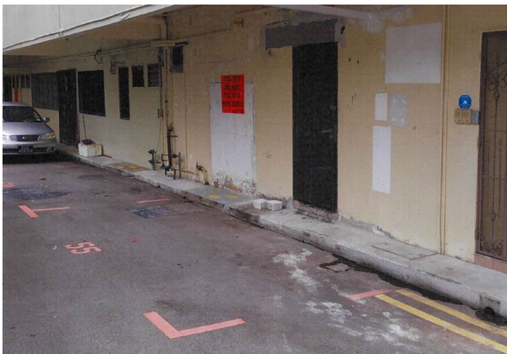
Figure 1: Current state of the rear of Unit 53
