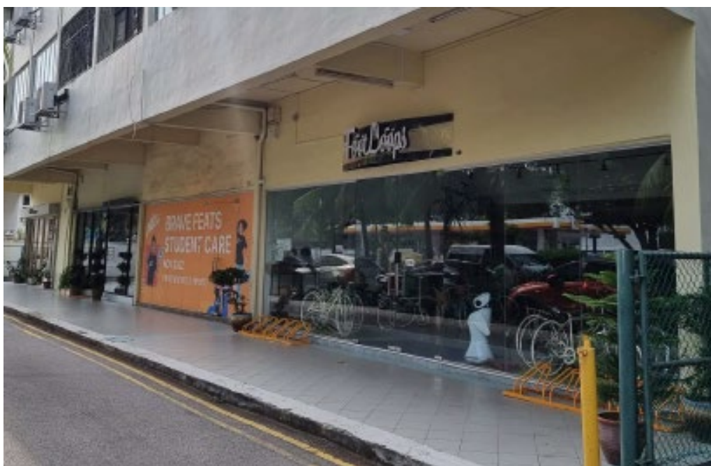
Figure 9: Photograph of the front of the Development from the right.
