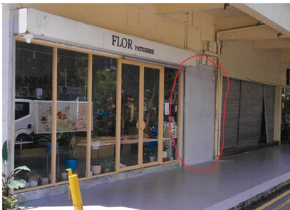
Figure 4: Side view of the front wall of Unit 53
